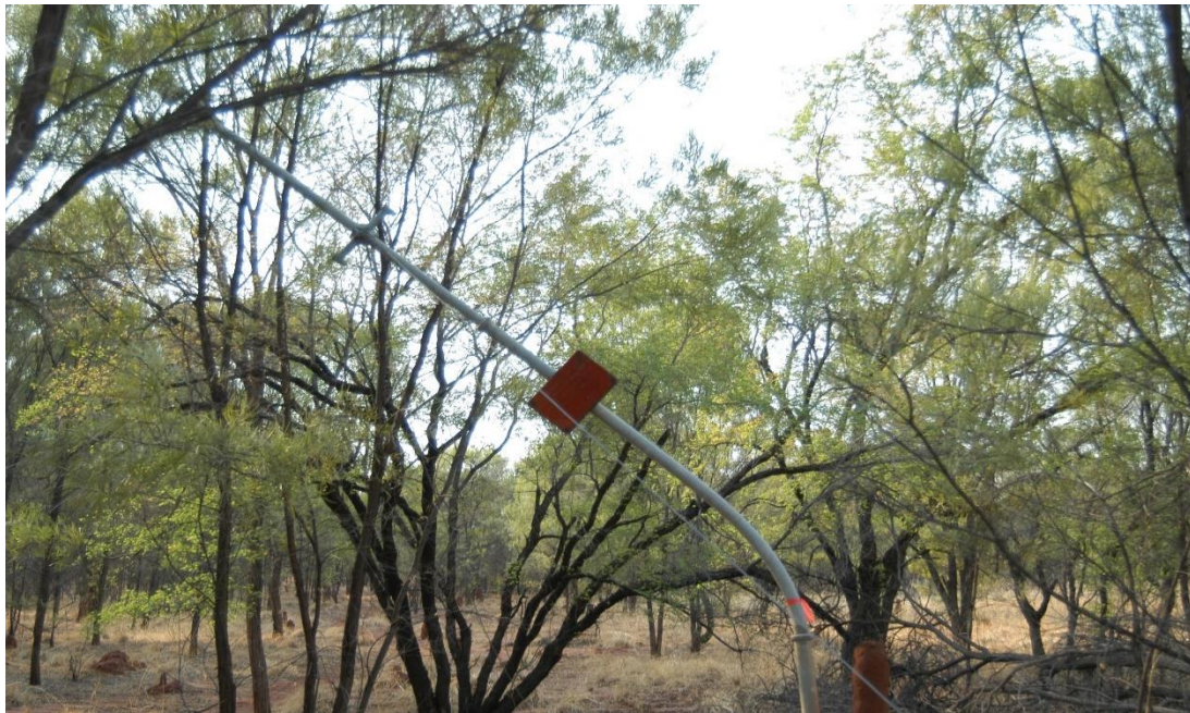
Joining Pole prior to the line being cleared and the pole straightened
