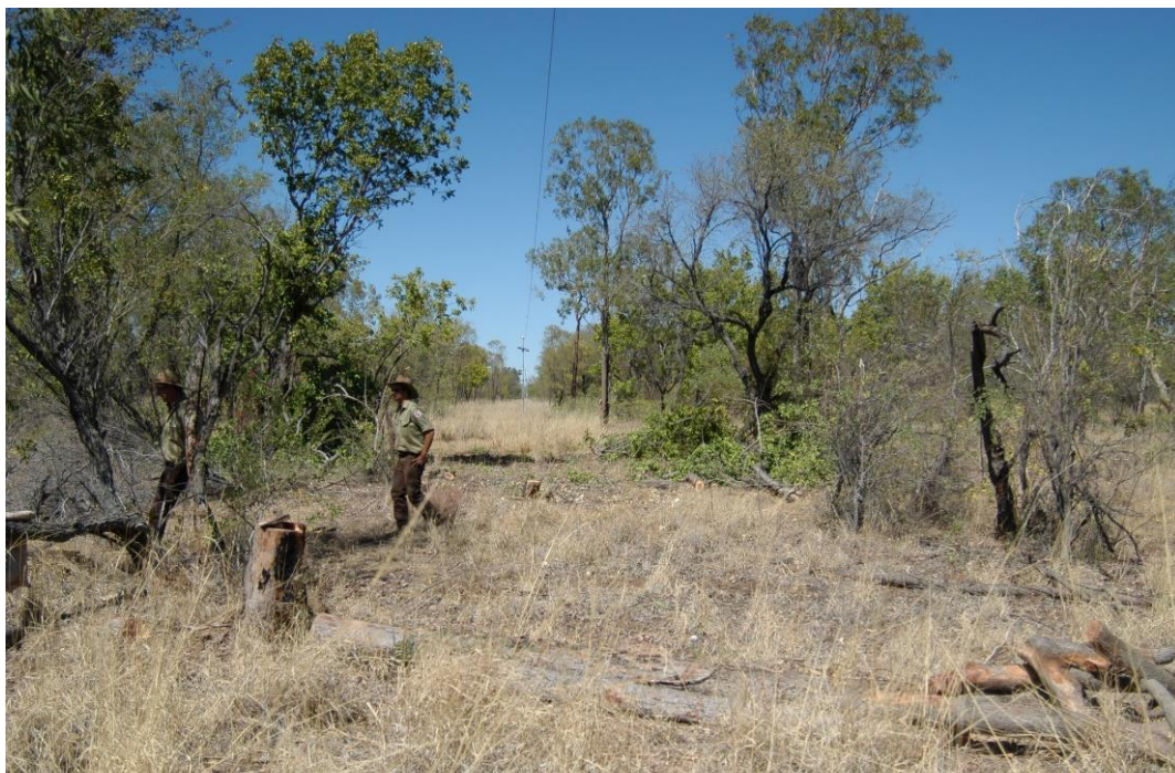
Line cleared and wire restrung southern end of reserve
